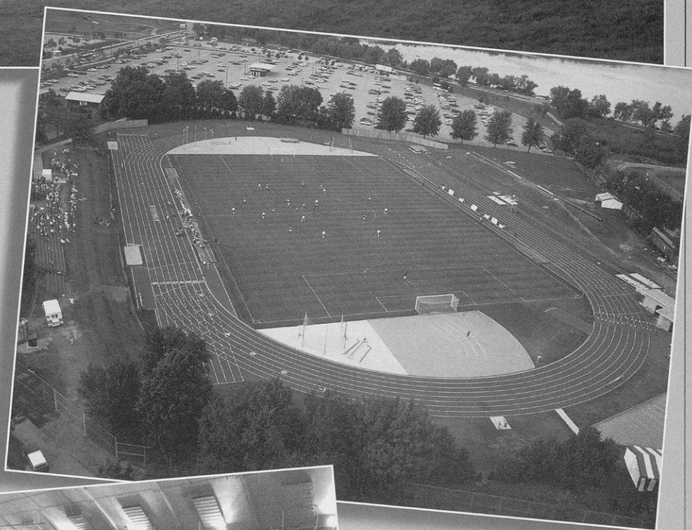
Right: The outdoor track and soccer complex, which is fully lighted, features a 400-meter Martin rubber surface with throwing and jumping areas in the infield. The soccer field is Olympic size and has natural grass.
